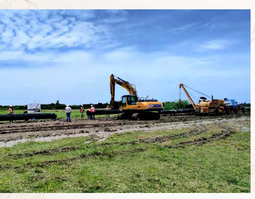
The process of lowering pipelines for transportation of petroleum products. IndianOil operates a more than a 15,000 kilometre long network of crude oil, petroleum products and gas pipelines. It is a pioneer in the country, managing one of the world's largest oil pipeline networks.
