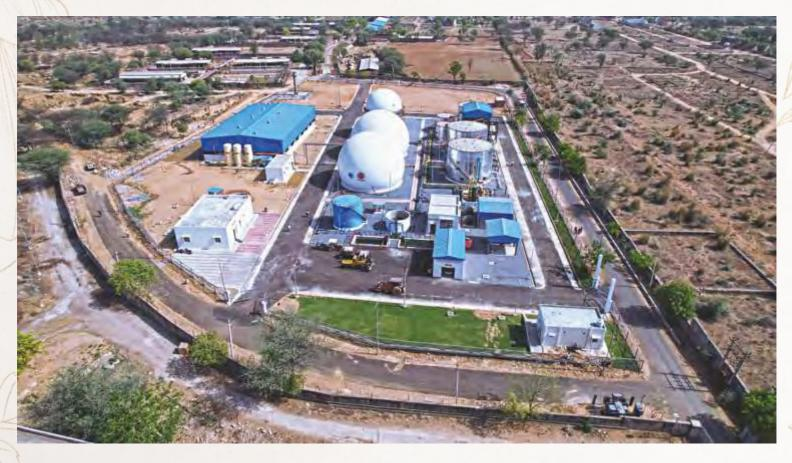
The IOT biogas plant which provides oxygen-free conditions for anaerobic digestion to occur. Simply put, it's an artificial system where you can turn waste into sustainable energy and fertilisers, with positive effects on the environment.
